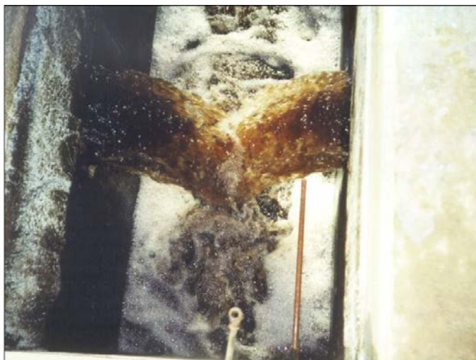
Figure 2: Typical backwash water after cleaning the filter media
