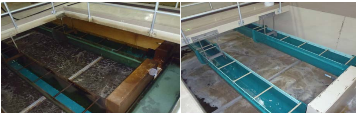
Figure 3: The spray-on/rinse-off chemical cleaning solution makes it easy to remove unsightly surface stains from filter basins.
